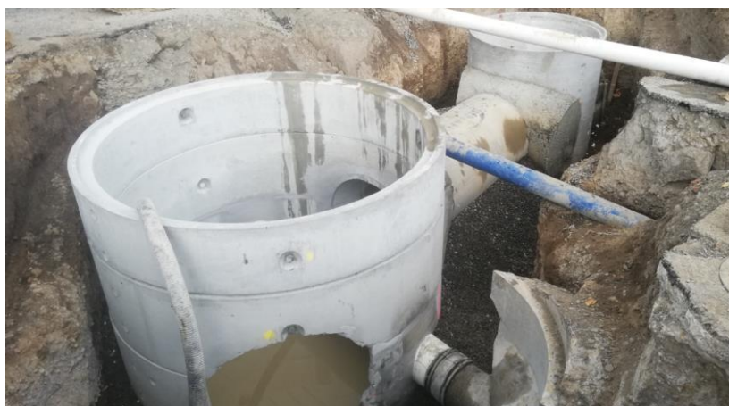
Installation of manholes on Francis Drake Street
