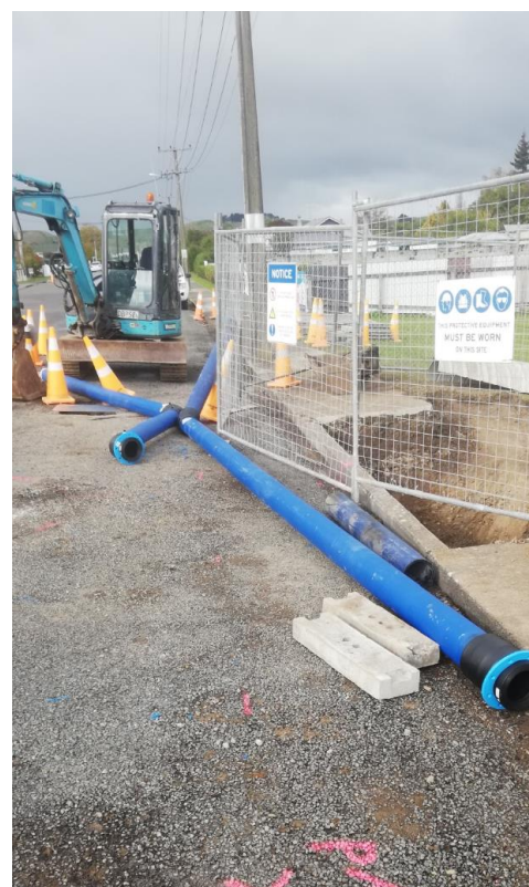
Relocate of water main on Francis Drake Street
