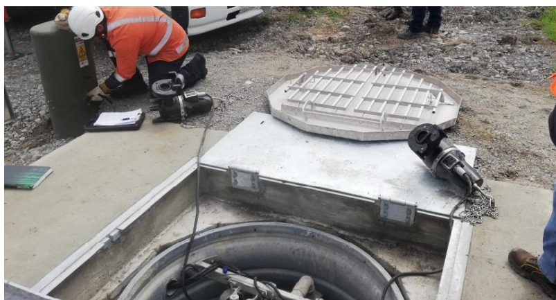
Technicians connecting pump station to power network
