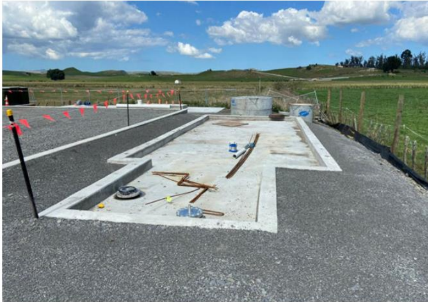
Figure 2: Otane Pump Station – awaiting pumps and pipework
