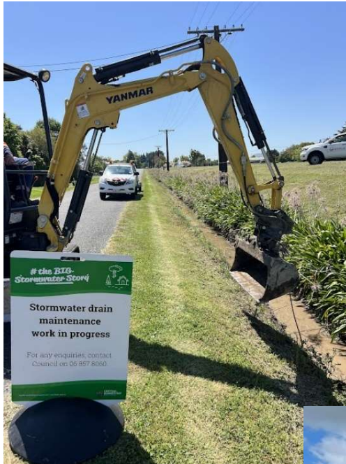
Figure 2: Minor excavation in Brogden St, Otane. Undertaken October 2024
