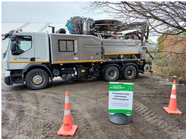
Figure 1: Pipe blockage clearance in Cook St, Waipukurau undertaken August 2024
