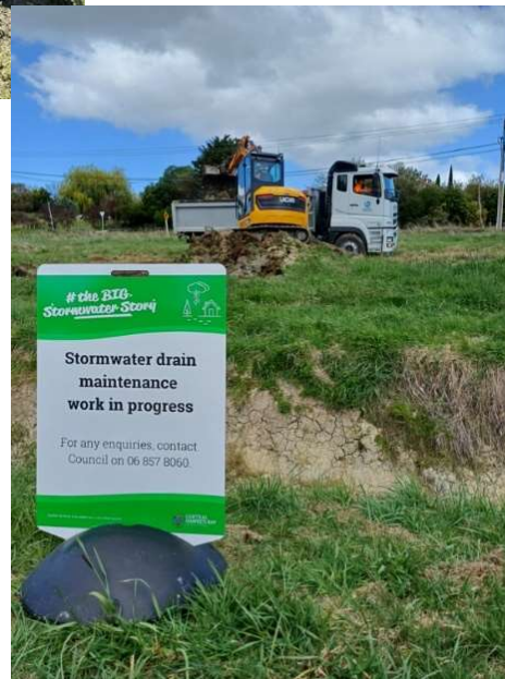
Figure 3: Major excavation in Watts St, Waipawa. Undertaken July 2024
