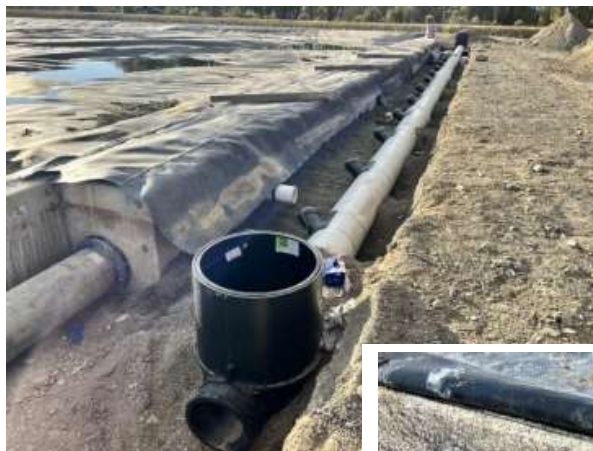
New manifold installation
