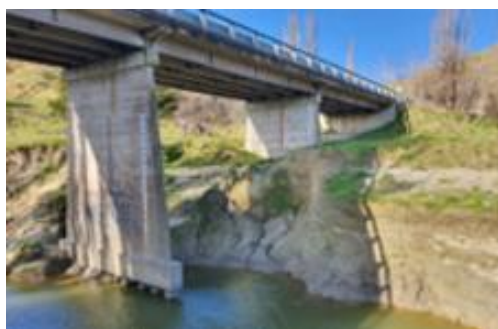
Wallingford Bridge- construction underway
