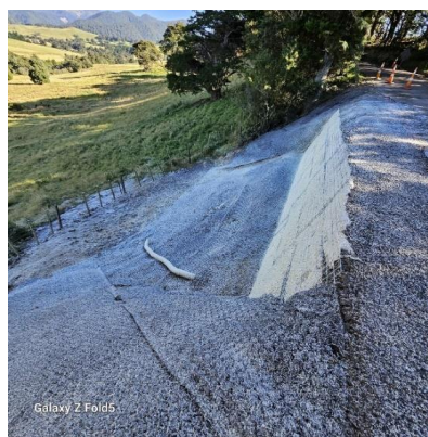
Wakarara Rd 28.4- work complete
