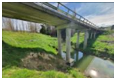
Renalls Bridge- construction to start 11 March
