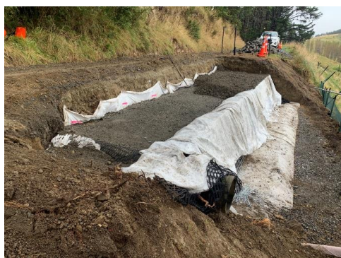
Old Hill Road 5.94- currently in progress
