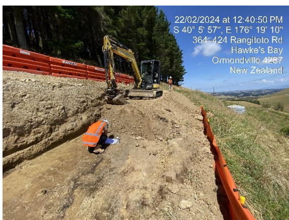
Rangitoto Road RP4.187- in progress
