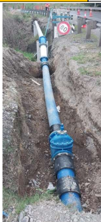
GREAT WATER UPGRADE TO (STAGE 1
