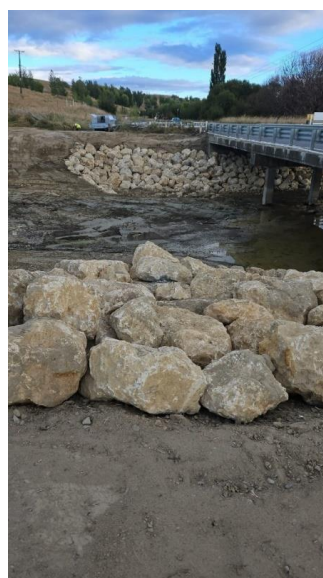
Flaxmill Bridge- nearing completion
