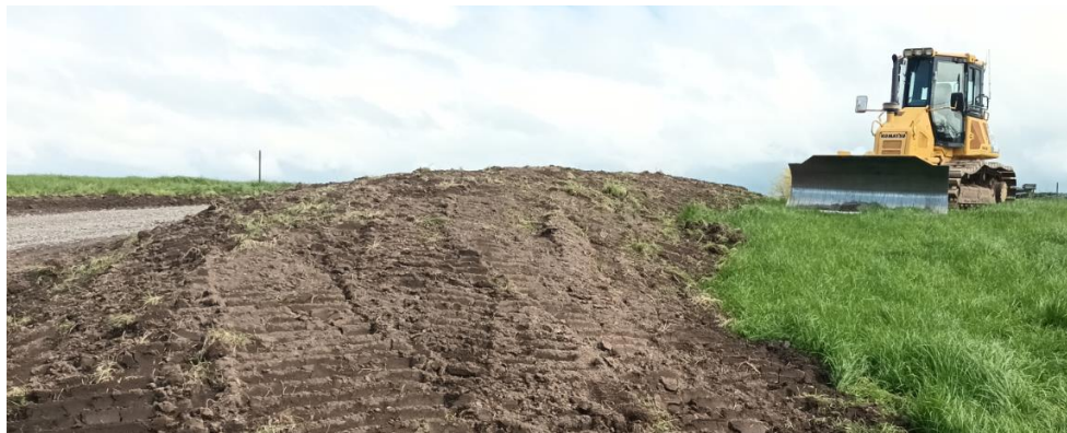
Figure 1: Bulldozer constructing access track to Eastern Interceptor Drain
