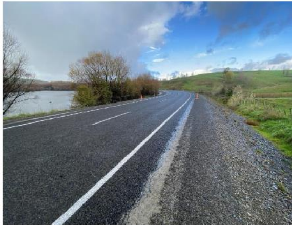
C1097 – Flaxmill Inundation Remediation Project (SP3): Basecourse testing, chipsealing and set out for road marking completed, guardrail installation and line marking commenced.
