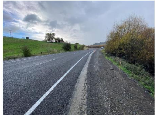
C1097 – Flaxmill Inundation Remediation Project (SP3): Basecourse testing, chipsealing and set out for road marking completed, guardrail installation and line marking commenced.
