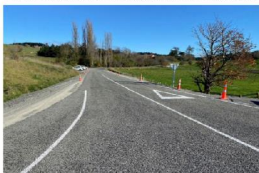
C1097 – Flaxmill Inundation Remediation Project (SP3): Basecourse testing, chipsealing and set out for road marking completed, guardrail installation and line marking commenced.
