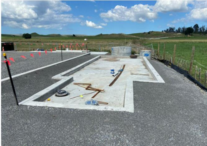
Figure 2: Otane Pump Station – awaiting pumps and pipework
