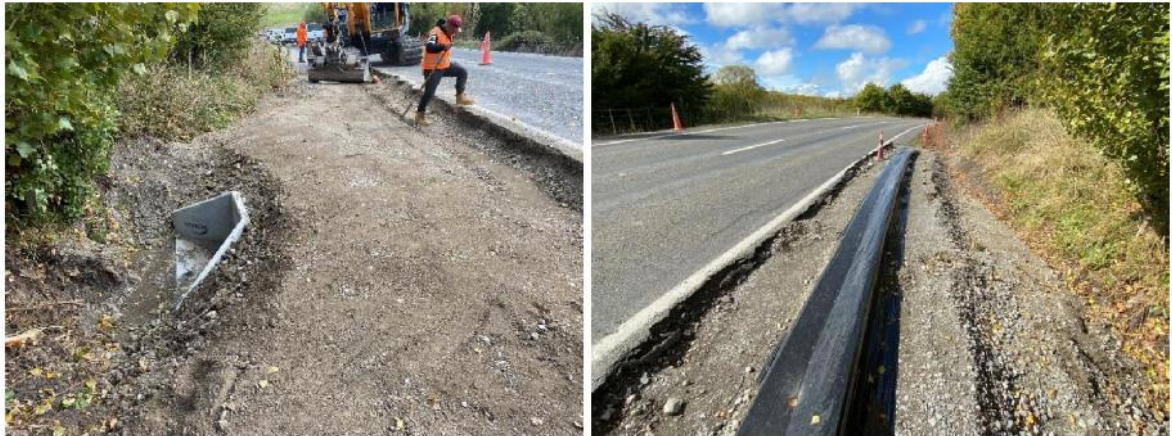
C1097 – Flaxmill Inundation Remediation Project – SP3: Basecourse placement &amp; cement stabilise at Porangahau Road
