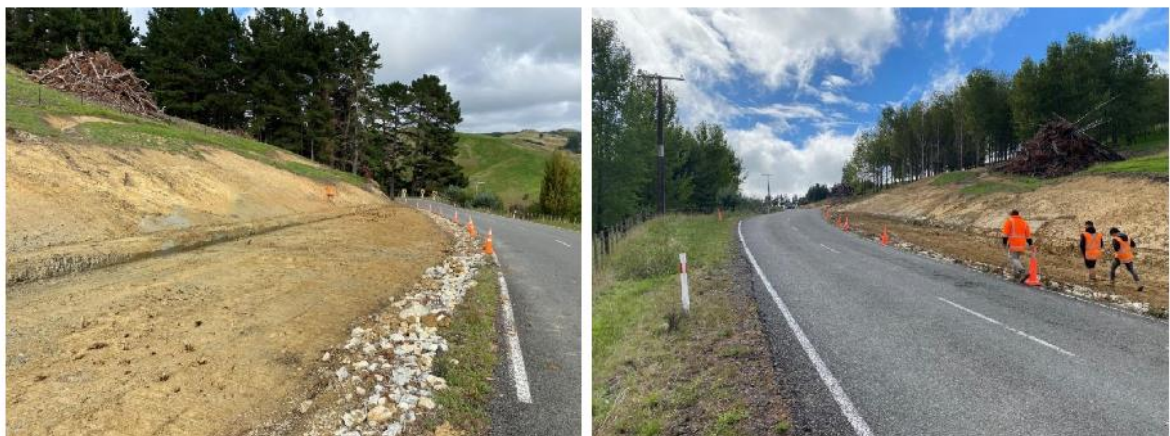
C1098 – Retaining Walls: Lower Wimbledon Retreat – Road excavation to subgrade complete, commencing installation of drainage
