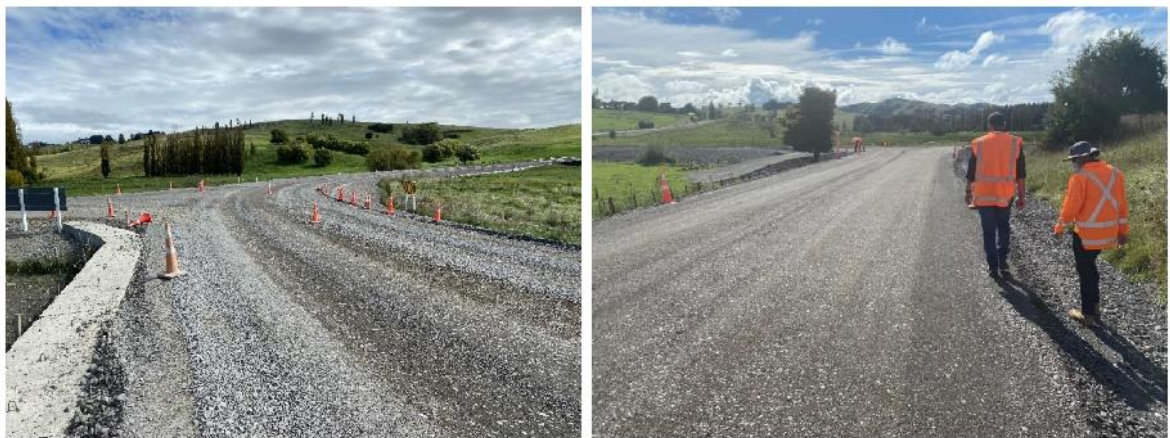
C1098 – Retaining Walls: Lower Wimbledon Retreat – Road excavation to subgrade complete, commencing installation of drainage
