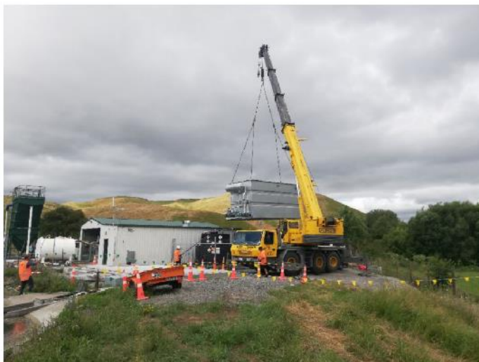
Figure 4: DAF unit craned into place
