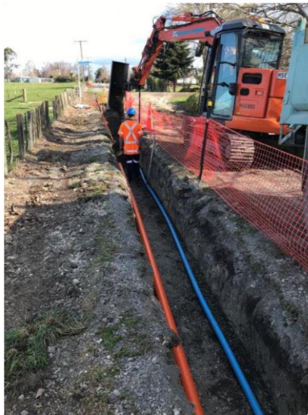
Co trenching service installation
