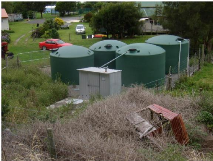
Figure 3-3 : Raw water tanks, spring and pumping station
