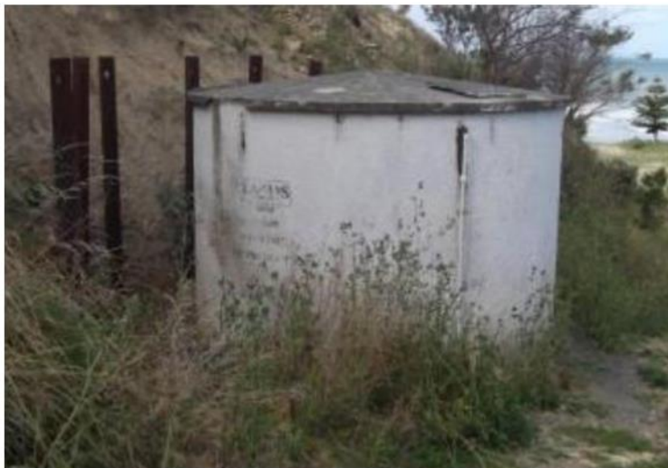
Figure 3-5 : Concrete treated water tank which supplies campground
