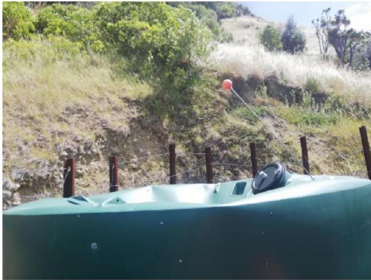
Figure 3-4 : Damaged treated water tank
