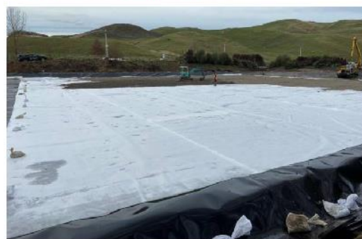
Preparation of the geobag area at Waipawa WWTP for desludging
