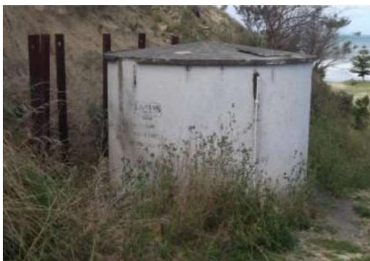
Figure 3-5 : Concrete treated water tank which supplies campground
