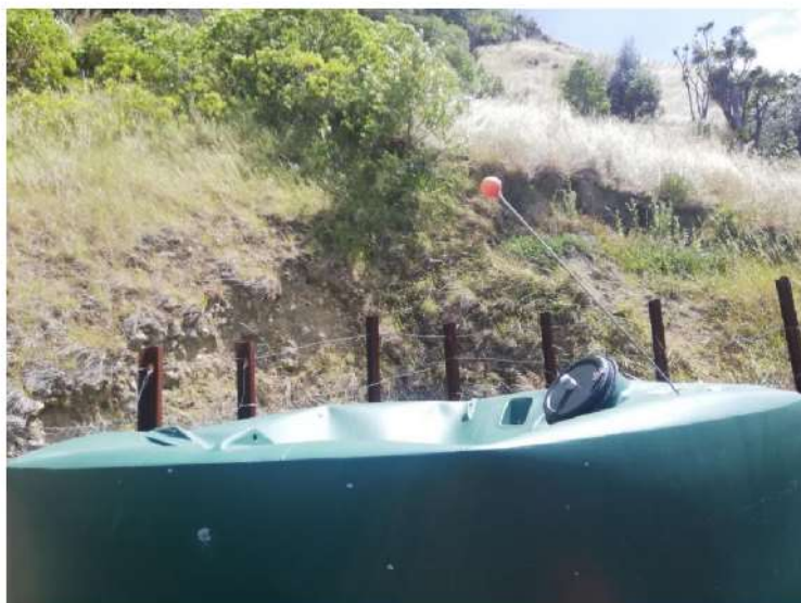
Figure 3-4 : Damaged treated water tank
